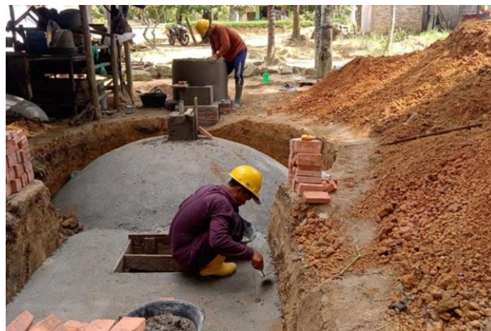
FIGURE 5. Biogas Reactor Manufacturing Process
