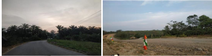
FIGURE 4. Road to Plumeria Eco Park
