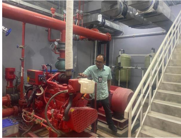
FIGURE 2. Inspection of the hydrant pump system during the preparation period
