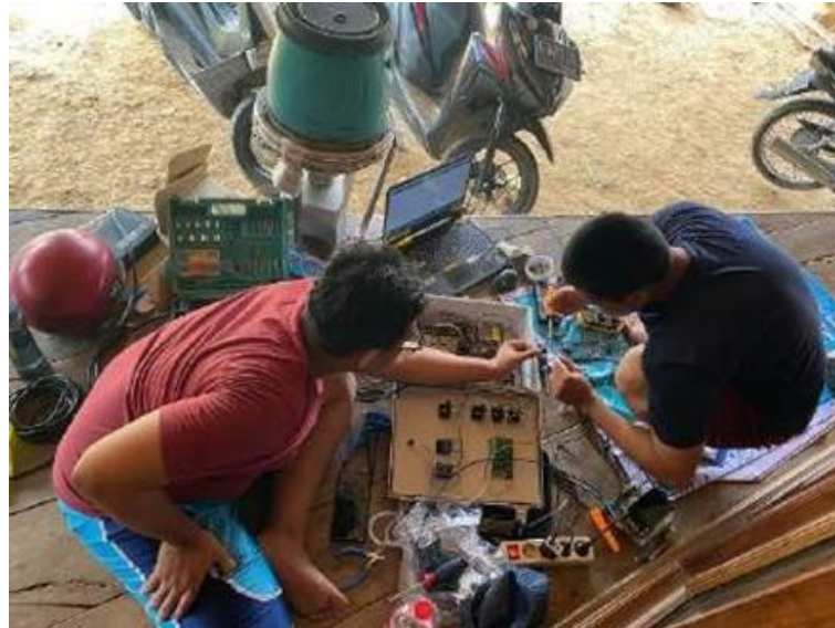
FIGURE 5. Control Panel Installation
