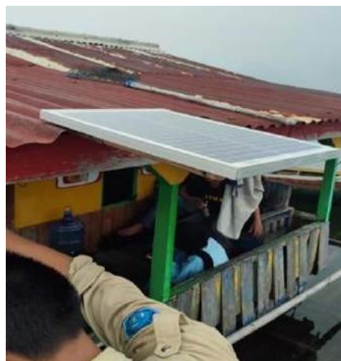
FIGURE 7. Solar Panel Testing
