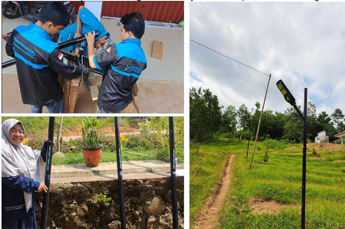
Figure 8. Solar panel lighting installation
