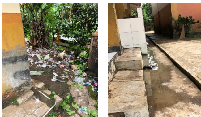
Figure 2. Condition of the Sukamanah II elementary school environment
