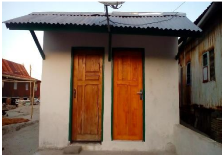
Figure 7. Public toilets on Kambuno Island, Pulau Sembilan
