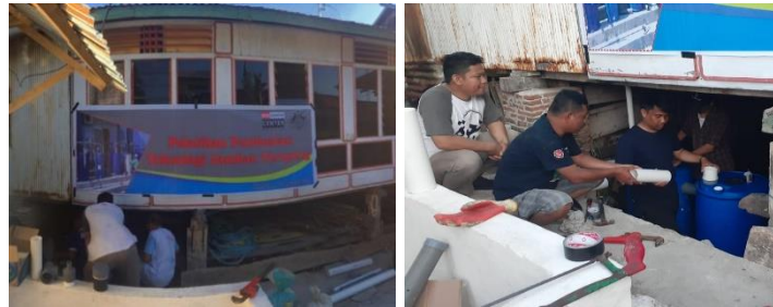
Figure 6. Assistance in installing Tidal latrines
