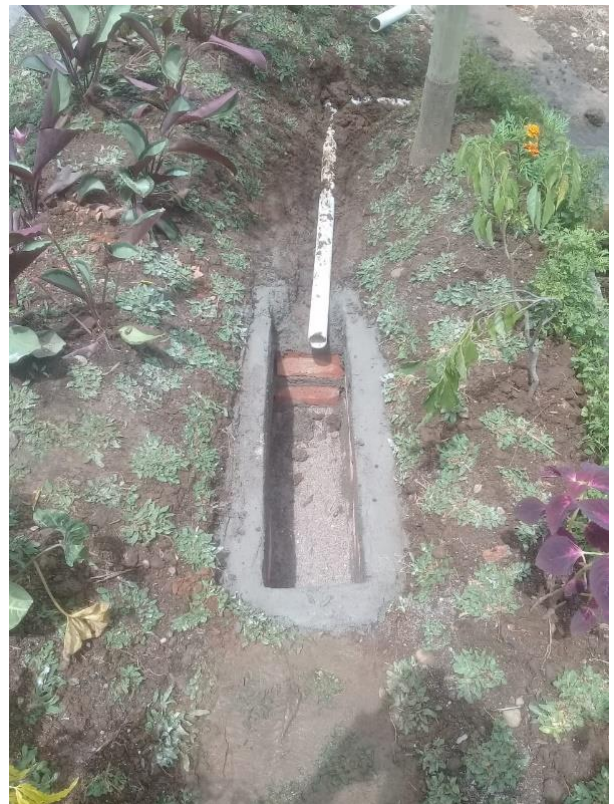
Figure 5. Rain garden equipped with infiltration wells at Ridho Residence
