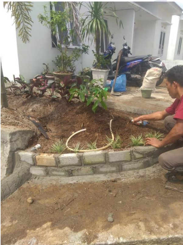
Figure 5. Rain garden equipped with infiltration wells at Ridho Residence
