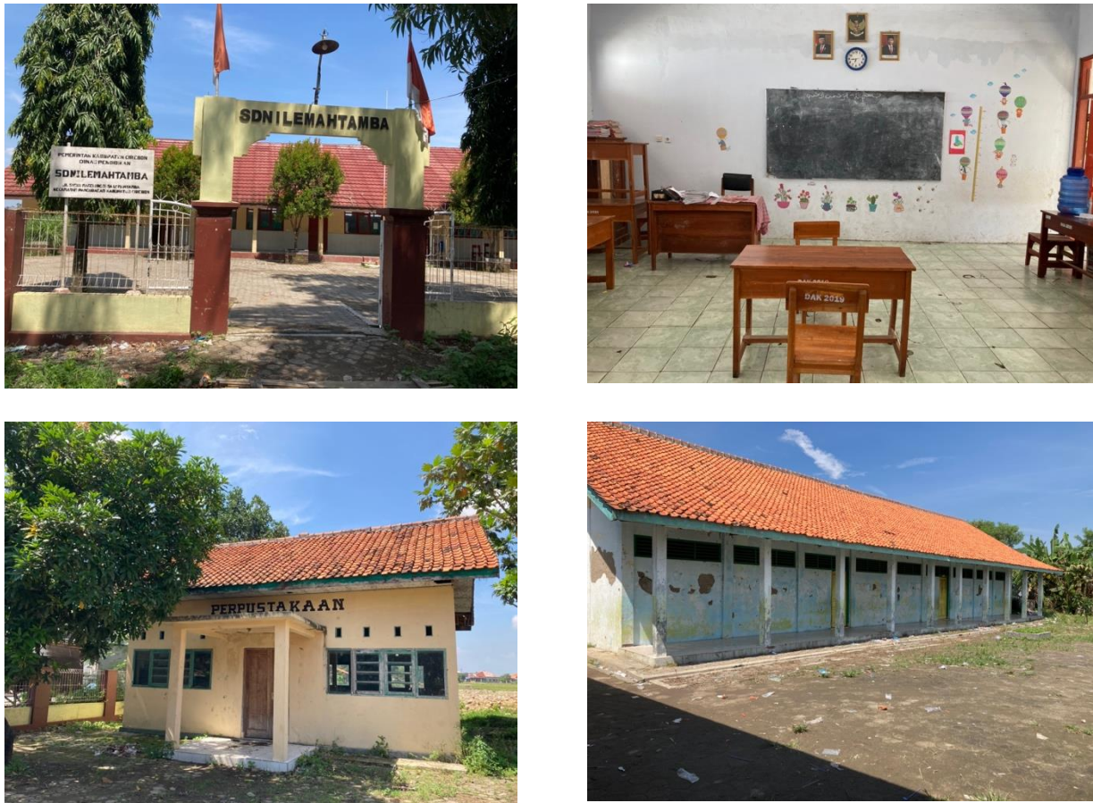
Figure 1. Condition of Lemahtamba 1 Elementary School
