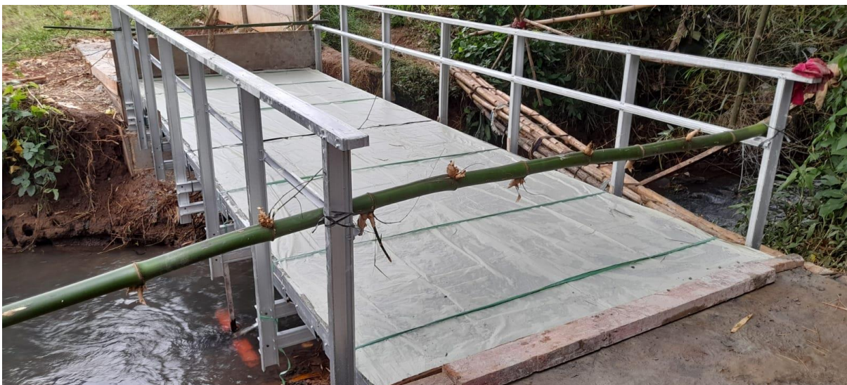
Figure 6: The span obtained from the bridge is 2 x 6 meters
