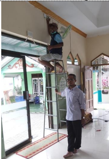
(a) Wifi Installation
