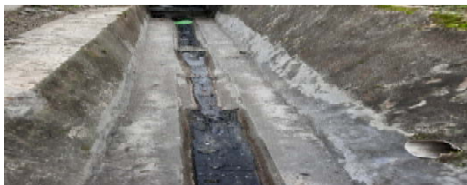
Figure 6. Implementation of drainage channel construction
