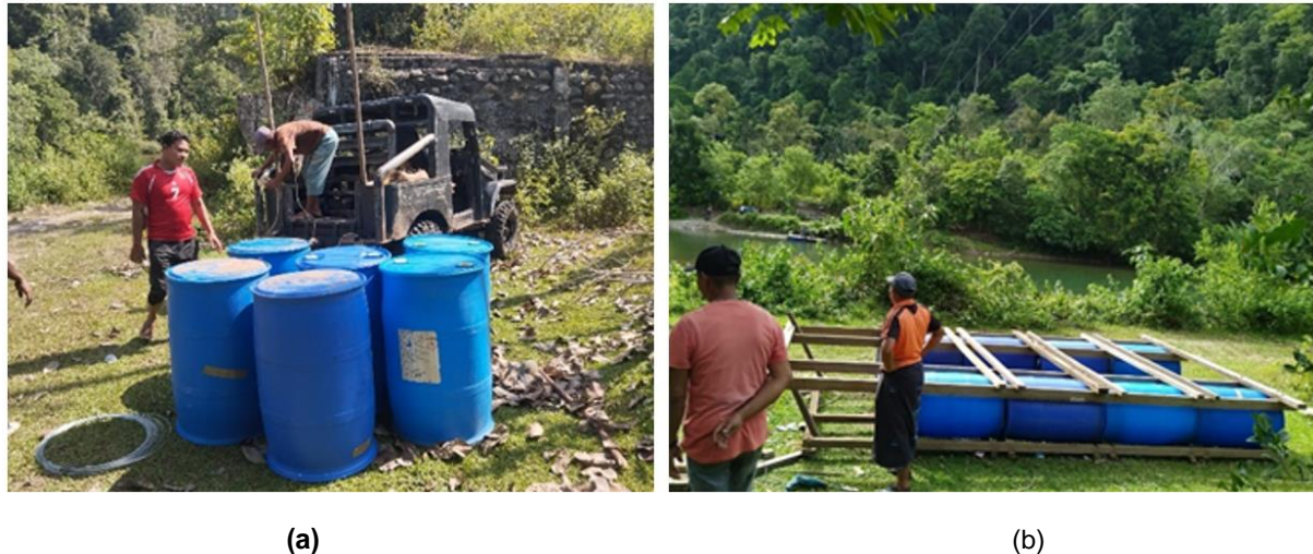
FIGURE 3. (a). Preparation of HDPE drums as flotation units. (b). The raft structure is formed by Integrating the drums into a timber frame
